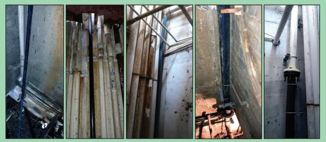
During the last couple of months, there have been multiple incidents of Riser pipe burst (from joints) causing stoppage of water supply at Towers for entire day or two as fixing of joints in PVC pipes takes long hours.
