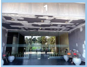
Due to seepage from ceiling and damages during maintenance from time to time, also because of prolonged wear & tear, Tower lobbies were in bad shape.
